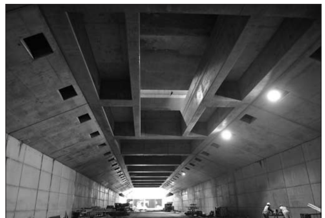
Fig. 9: Downward cross-supported reinforced concrete roof slab
