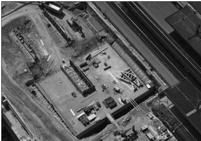
Fig. 8: Construction of the „U“ shaped eighth slab-bridge supporting three railway tracks
